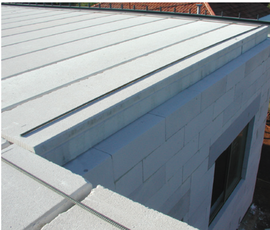
Image 7.3.2: Installed Floor Panels
