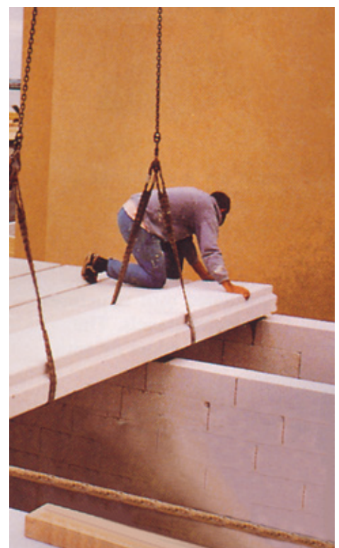
Image 7.3.3: Installing Floor Panels
